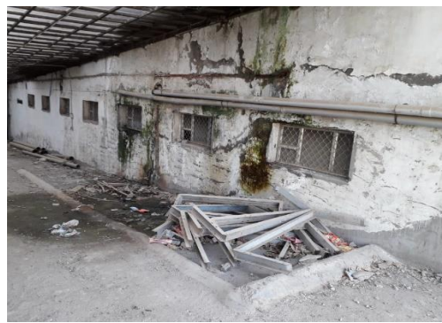
Water logging/seepage in basement of Research Hospital building
