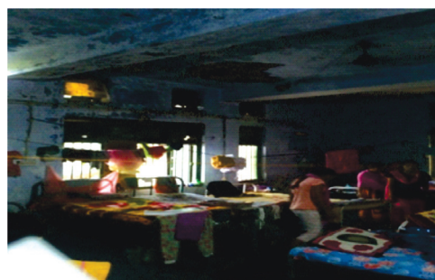
Hostel building of ANM School, Gaya
