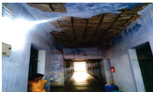
Hostel building of ANM School, Gaya
