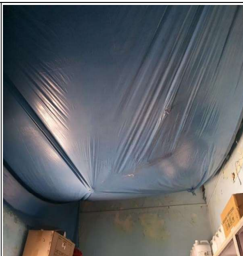
Plastic cover laid to protect from leakage in PHC, Kasoda, Taluka Erandol, District Jalgaon (17 March 2022)
