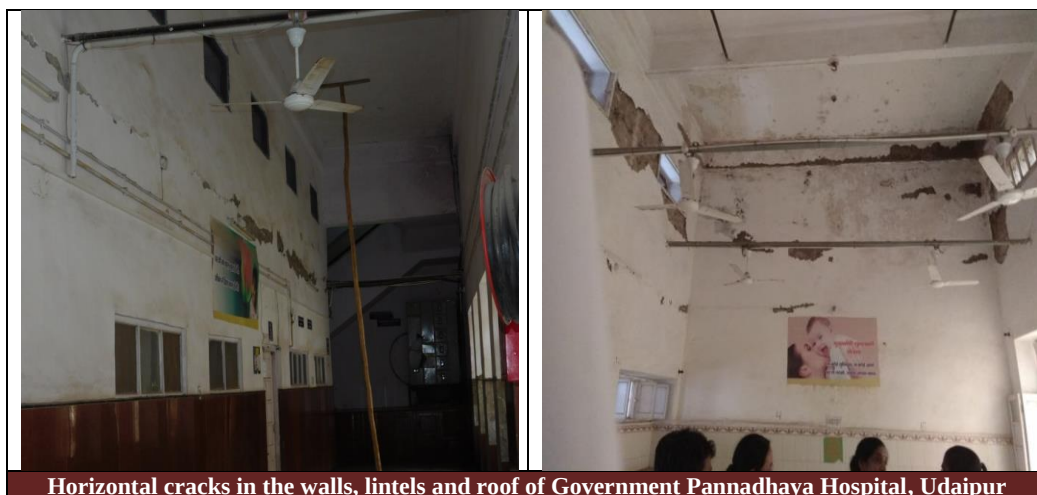
Horizontal cracks in the walls, lintels and roof of Government Pannadhaya Hospital, Udaipur
