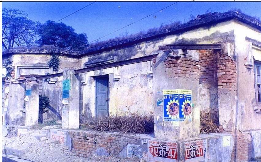
Building of PHC, Lalgang, Vaishali
