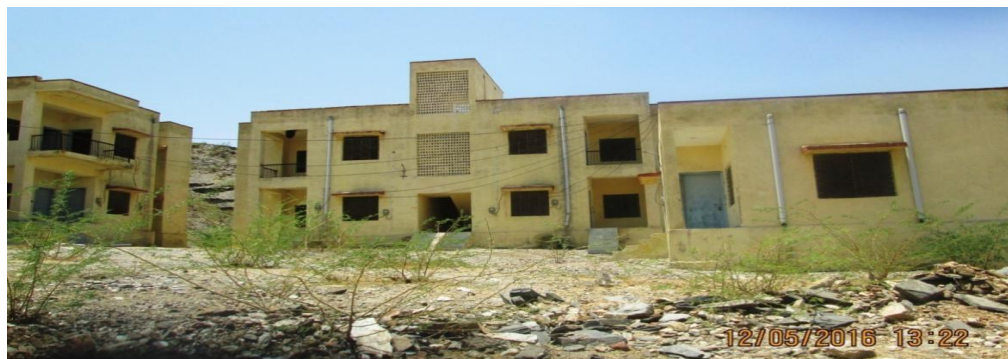
Unutilised Staff quarters at CHC Bhim, which were constructed 2.5 kms away from CHC building in an uninhabitable area.
