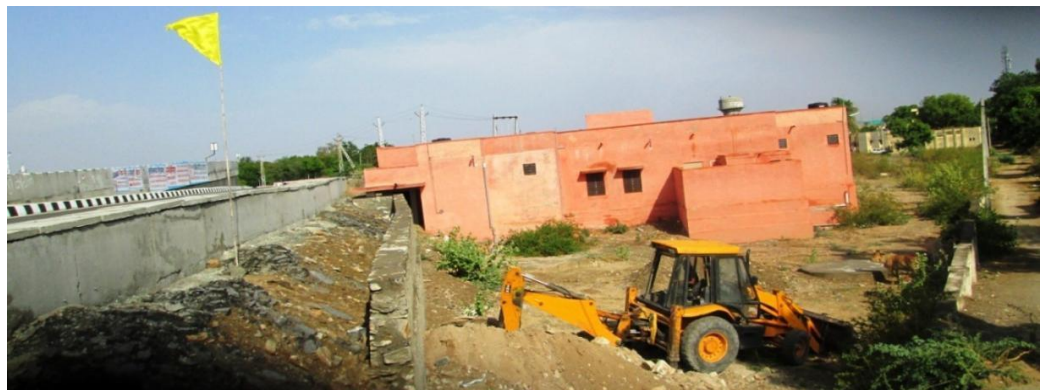
ANM hostel building at Rajsamand was constructed and was not utilised.
